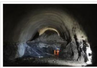
Drill+blast excavation progress
