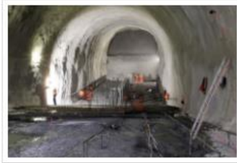
Works begin on the internal structures
