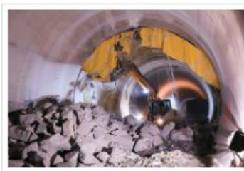
Works begin with breakout of the east tube lining
