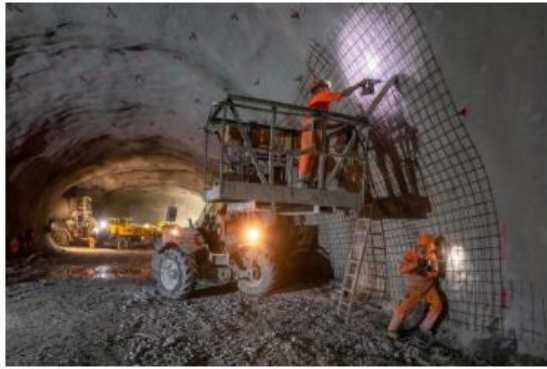
Primary support in the cavern topheading
