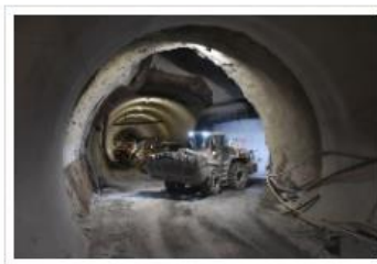
Mucking out into the main tunnel working area
