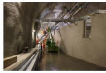
Settlement basin structure
